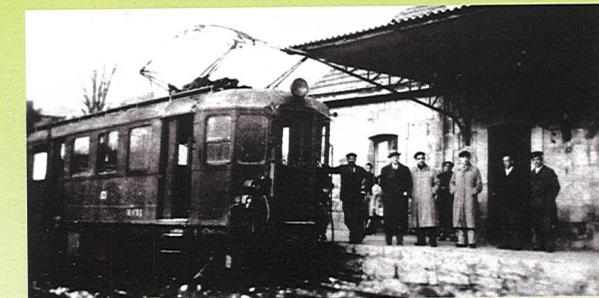
The Durango-Elorrio stretch was electrified in 1946, in a project designed by Italian engineer Lello Pontecorvo. This meant that all the rolling stock had to be changed. Passenger numbers increased substantially after this, and still further in the 1960s, then remained steady up to the closure of the line on 1 March 1975. The line was subsequently dismantled.
